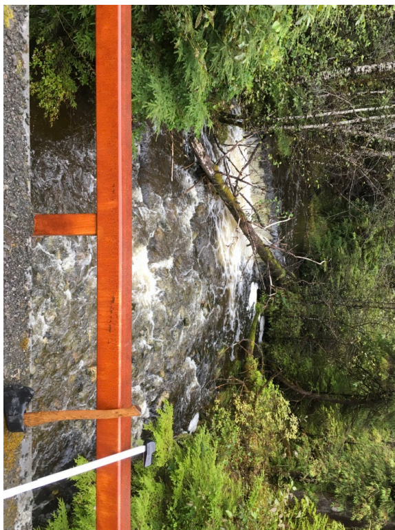
Upstream from Crossing
